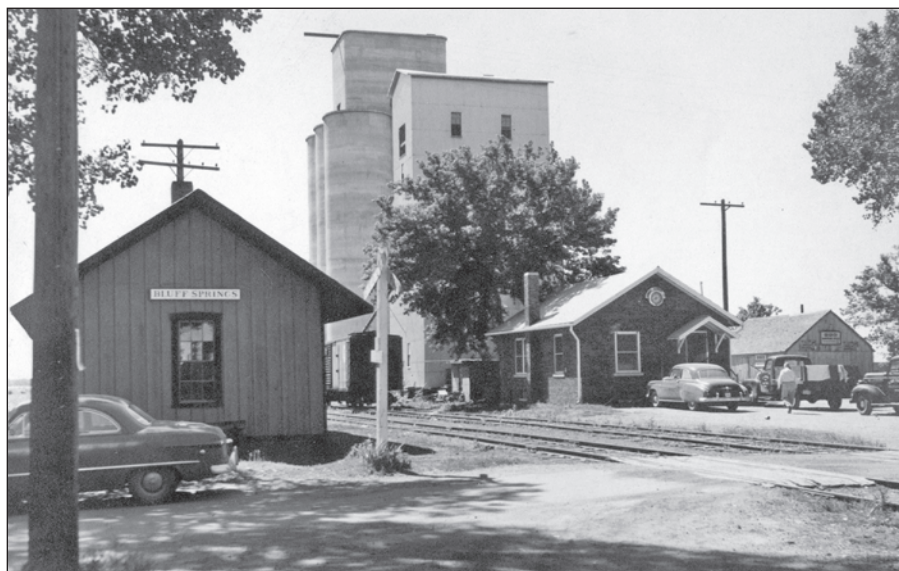
B&O's Bluff Springs depot as it appeared in the early 1950s.
